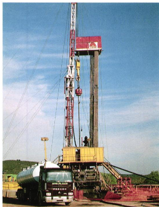
Plate 1 Drill rig on site
