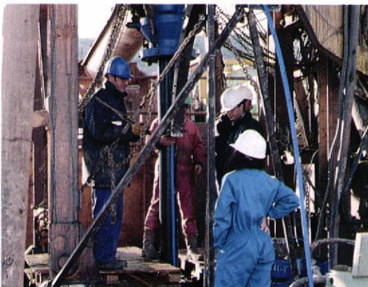
Plate 2 Attaching the instrumentation cable
