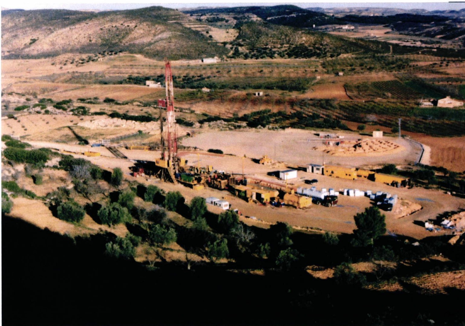
FIGURE 10 Production Well Drilling Works
